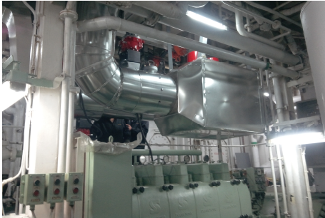
Fig. 2 Picture of SCR system in Kaya ship
